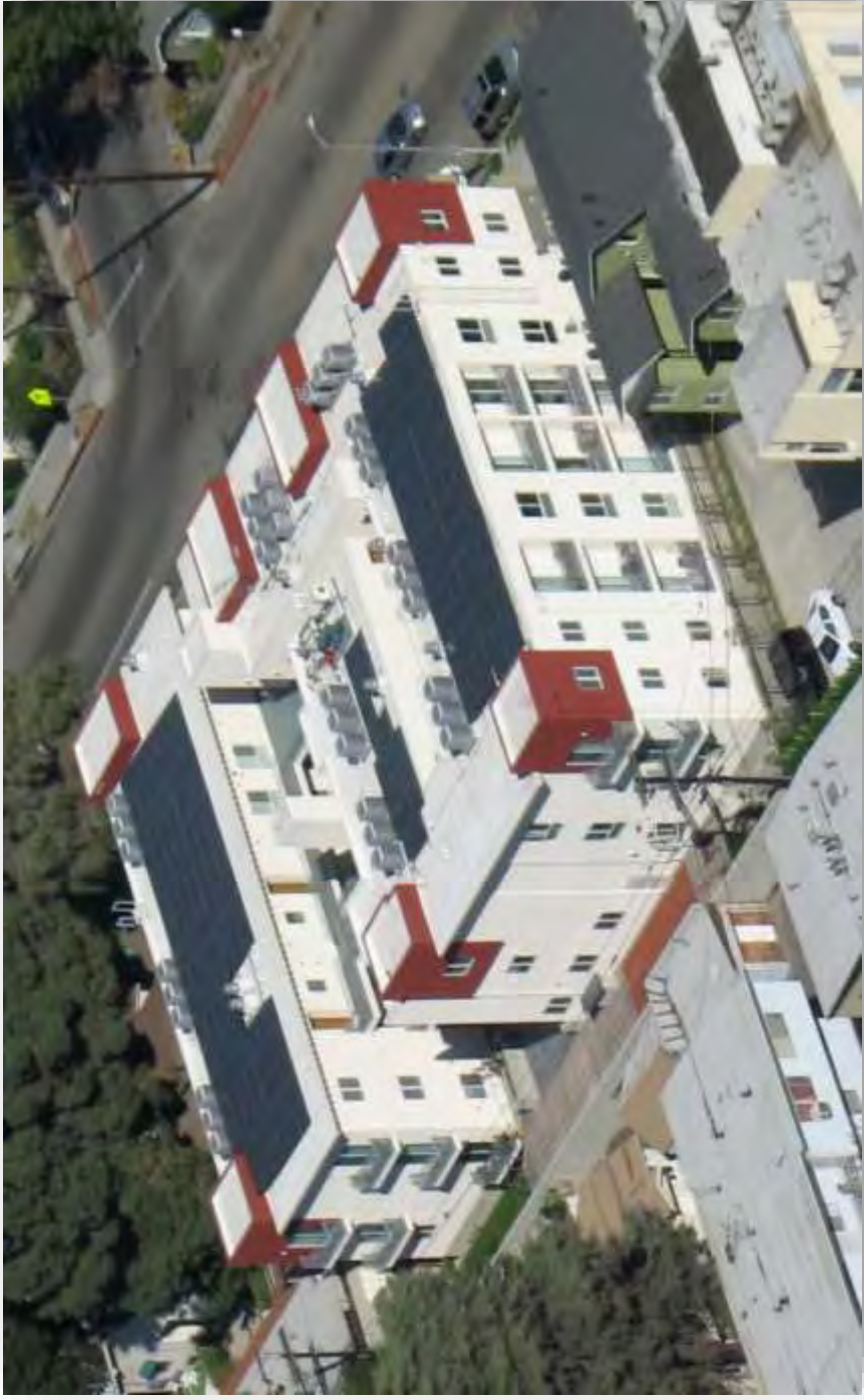
Affordable Housing 105 Units LEED Gold Certified Bronson Court Apartments, Los Angeles, CA
