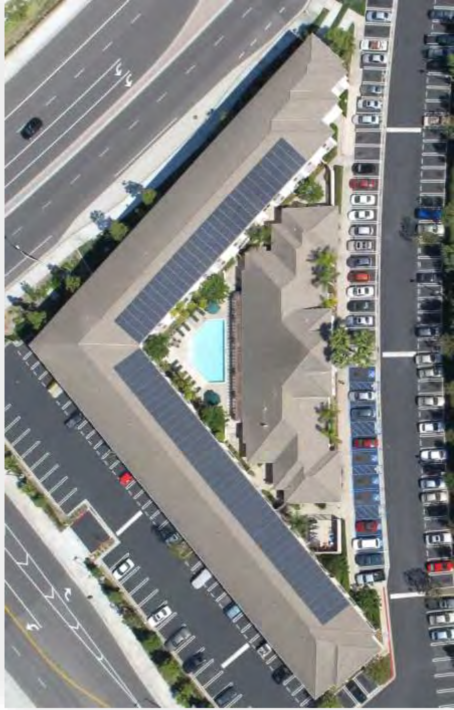
Irvine Inn Affordable Housing Project Irvine, CA
