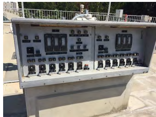
Right: Electrical/Instrumentation Upgrades
