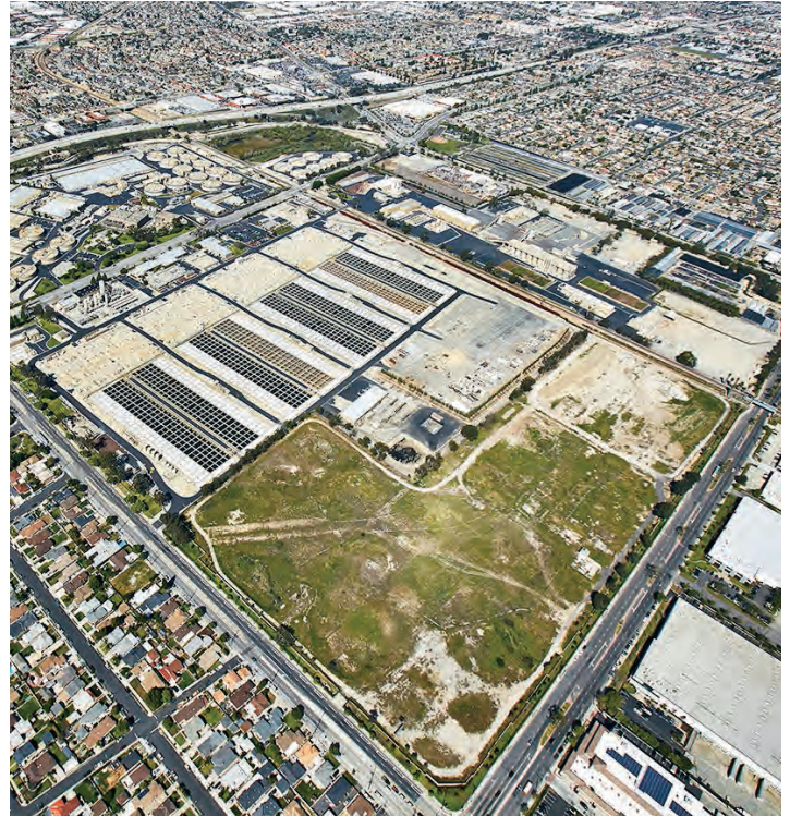
Sanitation Districts’ Joint Water Pollution Control Plant in Carson
