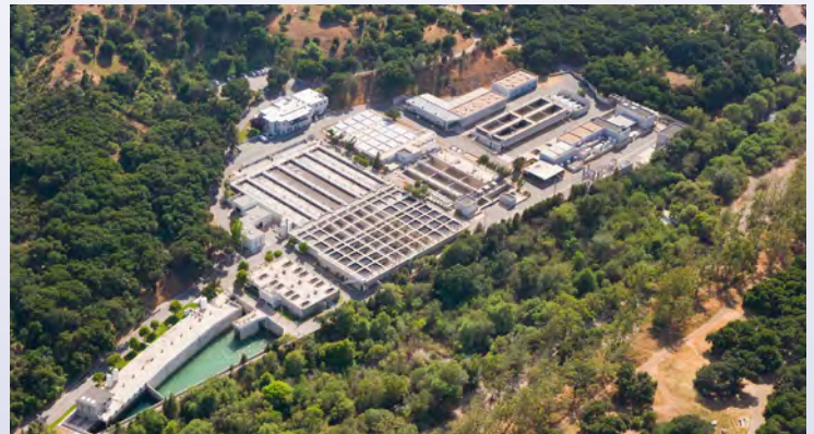
Built in 1965, each day the Tapia Water Reclamation Facility treats upward of nine million gallons to Title 22-Tertiary Treated Recycled Water standards.
