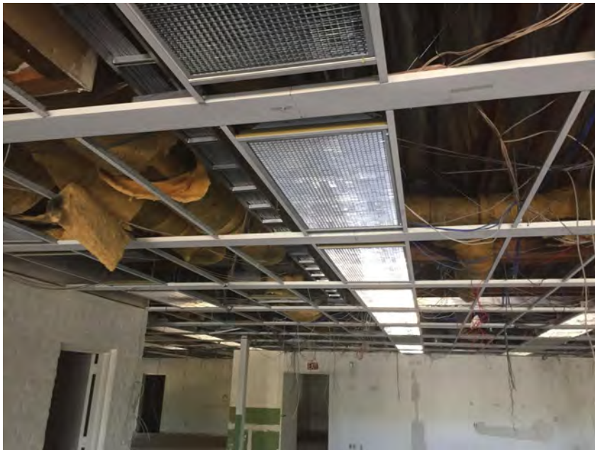
Figure 2-6 Typical Office Ceiling
