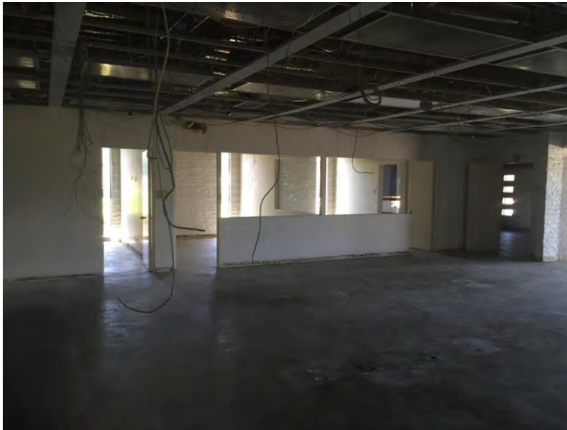
Figure 2-7 Existing Building Office Space
