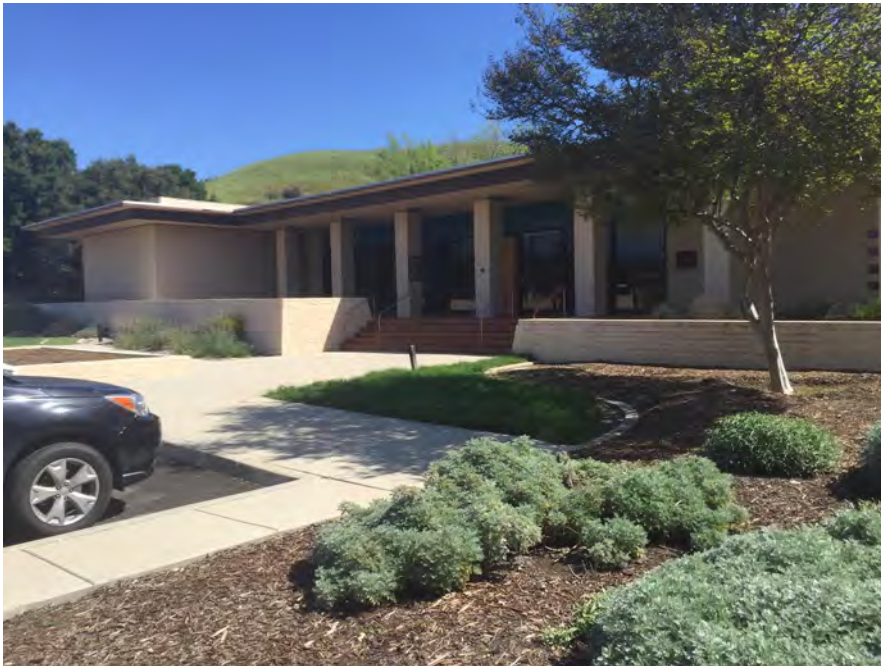
Figure 2-2 Existing Building Front Entrance (west side)
