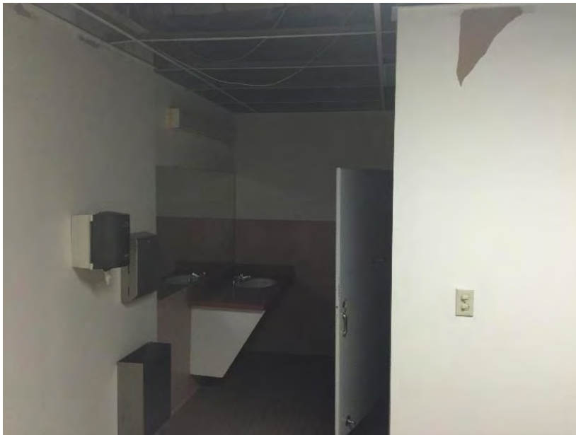
Figure 2-9 Existing Building Restrooms
