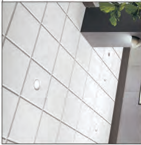
2X2 WHITE ACOUSTICAL CEILING TILES
