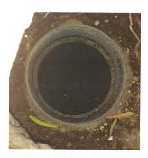
The above photo shows what our septic hole looked like on 10/02/15, after it had been fully pumped. When the plumbing company came this hole has been filled to the top with water, affecting our leaching system. After the pumping, it was completely empty. In less than a week, it was already filling up again.
