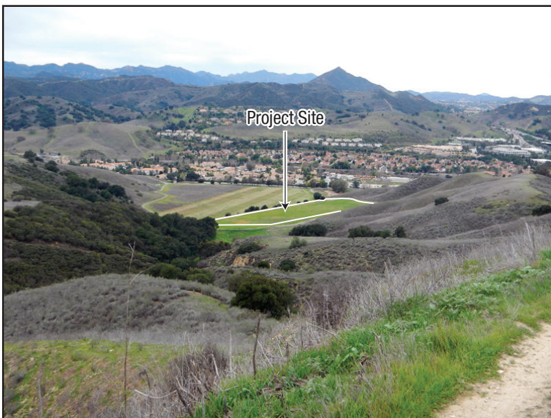
View 3 Westerly view of the project site as seen from the New Millennium Loop Trail, showing residences and commercial development of western Calabasas. Photo taken February 2, 2013.
