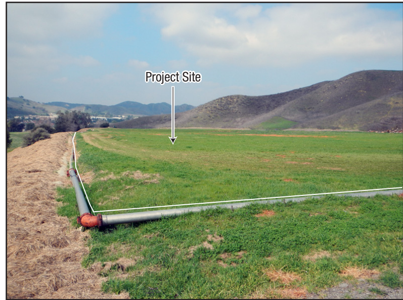
Photo 1B - View to the southeast of the upper field at the proposed solar site.
