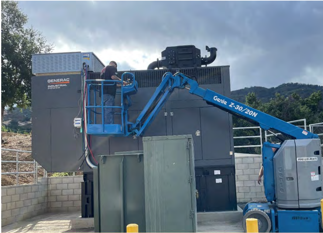
Figure 3 - Completing installation of 500 kW generator at Seminole Pump Station
