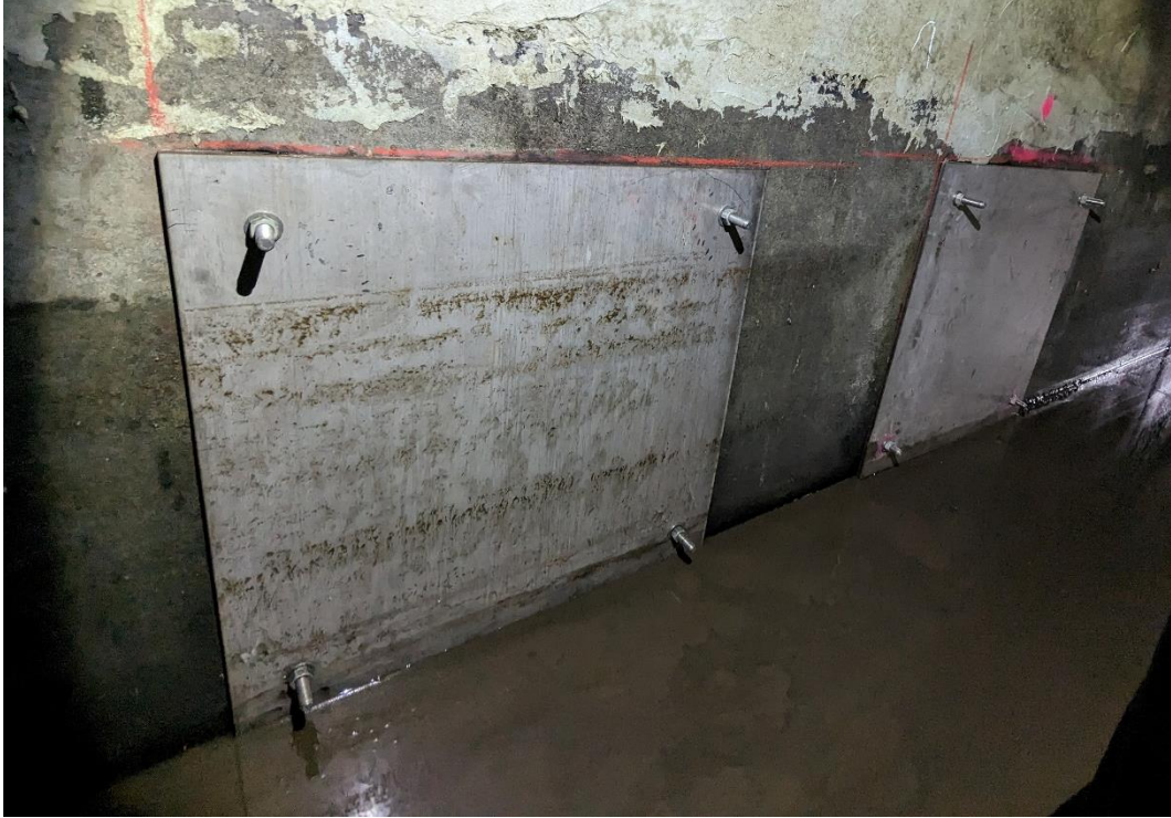
Figure 1-Stainless steel plates installed in Channel No. 2
