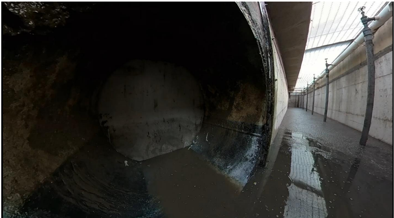
Figure 2-Selector Channel side of stainless steel plates, before cleaning and concrete infill.
