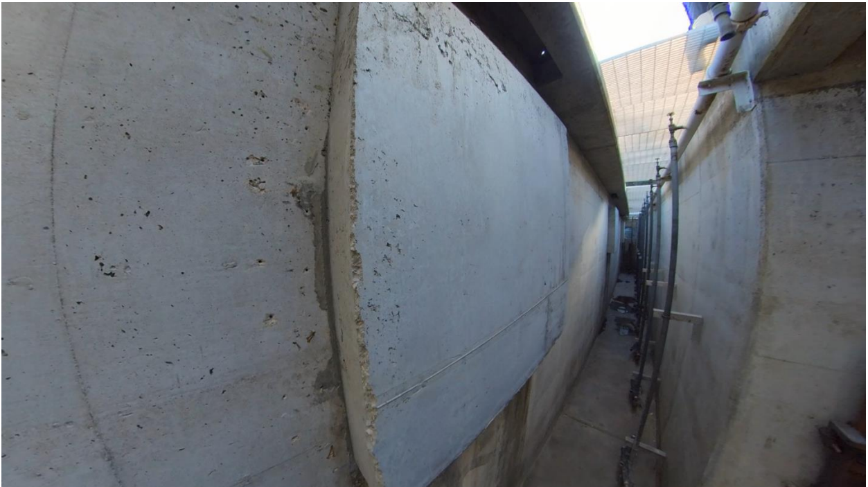
Figure 4- Completed concrete wall infill in selector channel.
