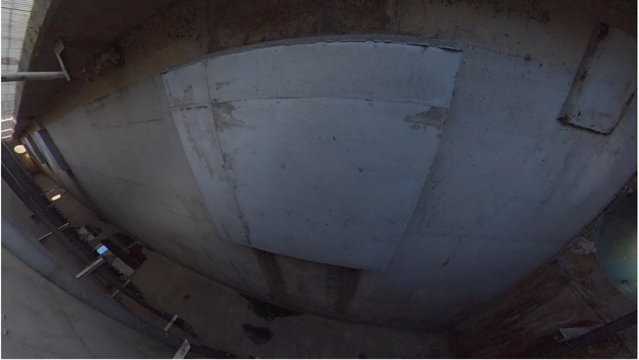
Figure 3- Completed concrete wall infill in selector channel.
