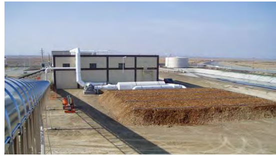
South Kern Compost Manufacturing Facility. Synagro utilizes an enclosed biosolids receiving and mixing building along with biofiltration in its compost system that controls VOCs and odors for the surrounding area.
