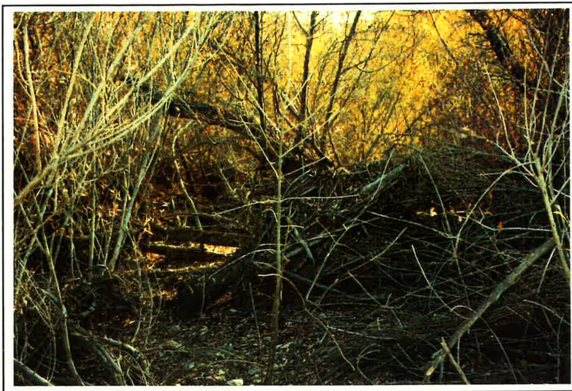
Figure 4.6 Debris Blockage Caused by Willow Growth
