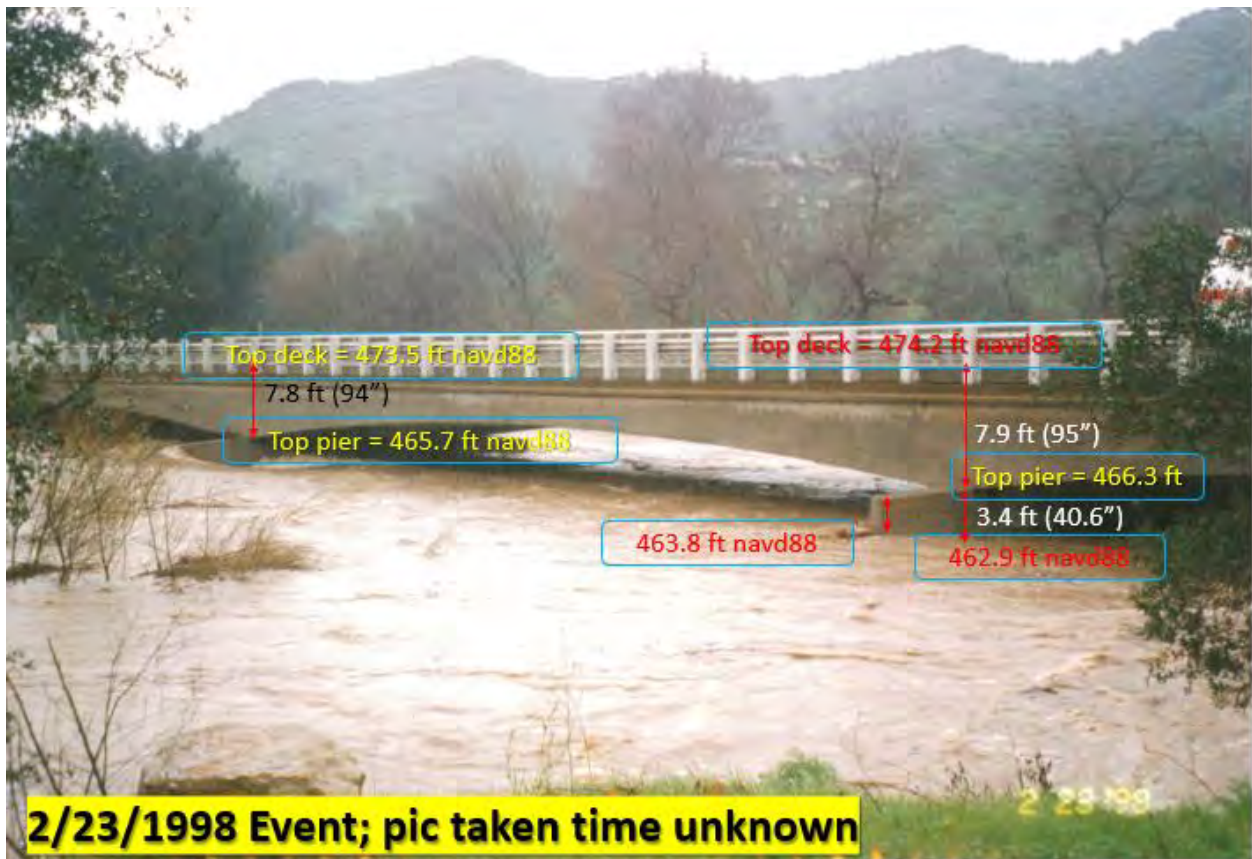
Figure 13 Water Level Estimation of the High Water Marks at the Malibu Canyon Road Bridge during the 12/30/2021 Flow Event and the 2/23/1998 Event (Note: The 2/7/1998 flow event was greater than the 2/23/1998 event, the available HWM during the 2/23/1998 was used as a substitute.)
