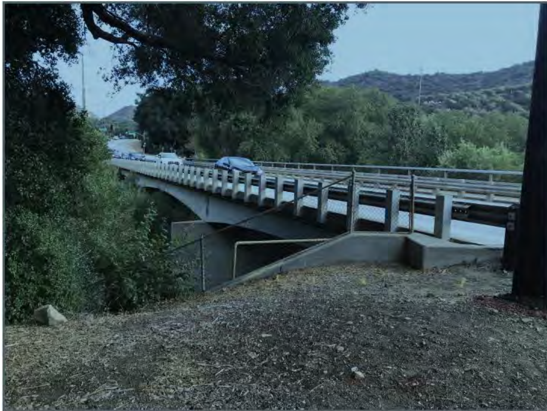
Photo of Malibu Canyon Road Bridge Taken on 9/14/2022 (Looking North)
