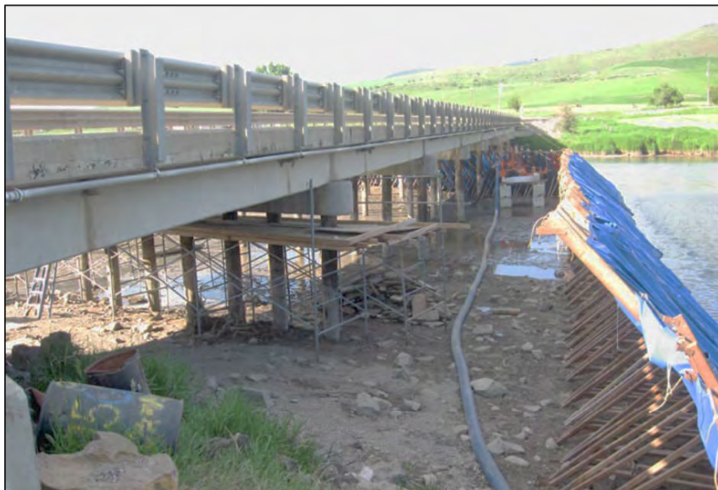
b. Example installed cofferdam system
