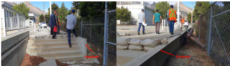
Photo of the Downstream Segment of the Existing Floodwall
