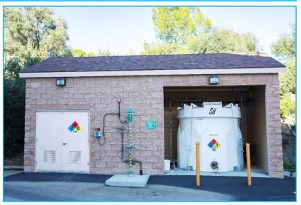
The El Toro Water District (ETWD) existing 2MG and 3MG potable water tank reservoirs had difficulty with chlorine residual due to temperature stratification. ETWD contracted PACE to design new tank mixing systems with a residual sampling system, a liquid chemical injection system and storage facility, and a new building with automation and site security. Civil, mechanical, electrical and
