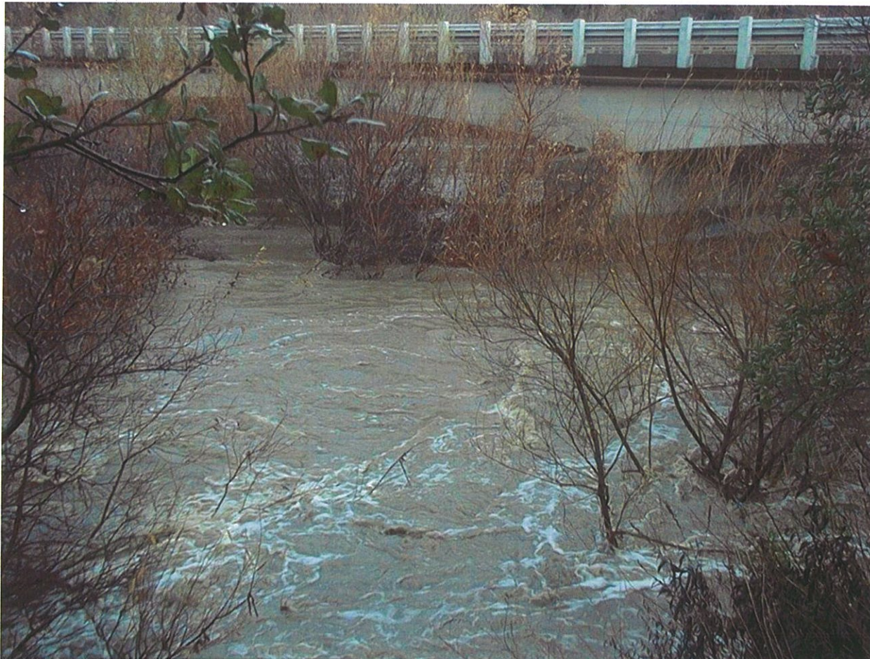
January 10, 2005 Malibu Canyon Bridge top of the pier is at elevation of 465 feet. Peak Flow 12,700 cfs.
