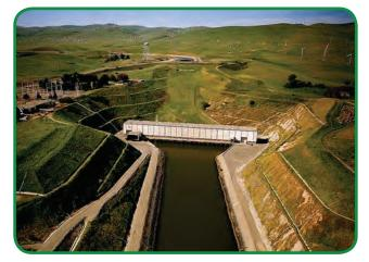
At the south end of the Delta, powerful pumps lift water into the California Aqueduct, continuing its journey south through California's Central Valley.
