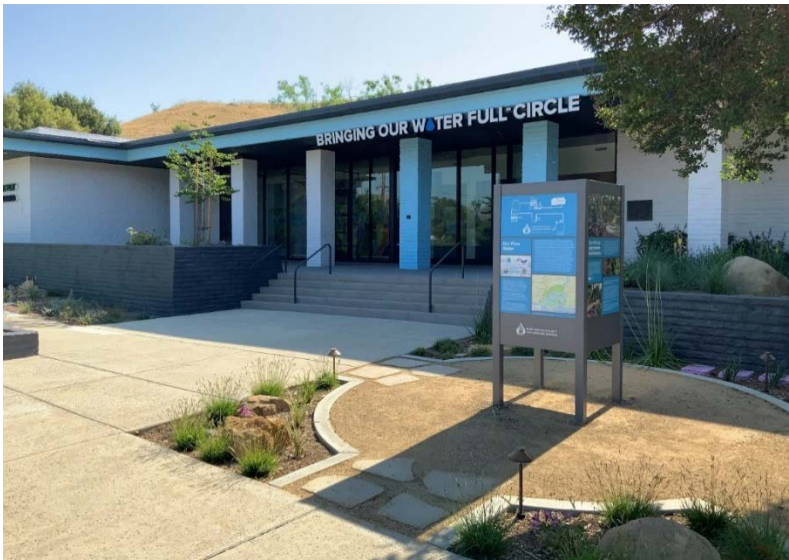
Figure 1 Exterior of LVMWD Pure Water Demonstration Facility.
