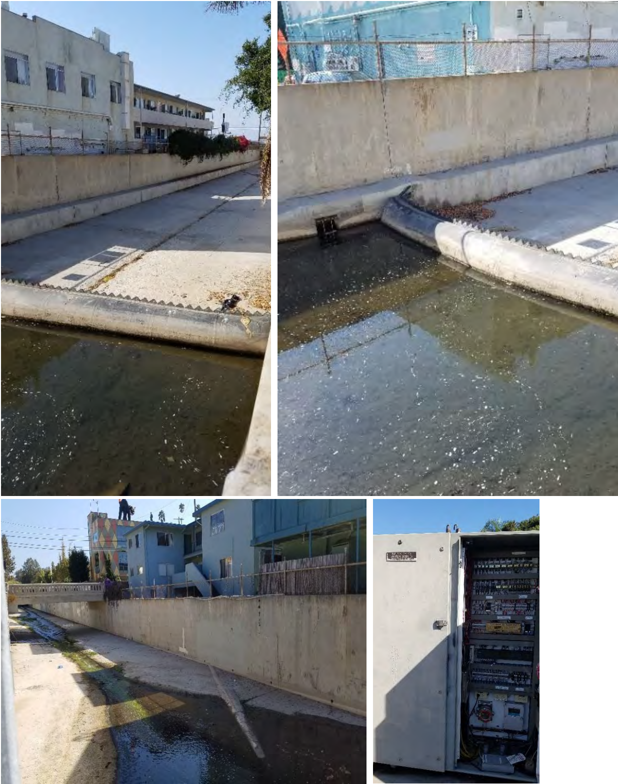
Photo 3-3. Santa Monica Canyon DWD; Photographs taken during October 15, 2019 Site Visit with LASAN Staff
