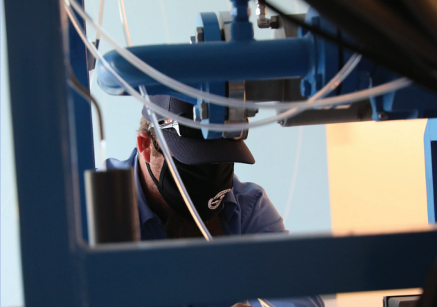
Burt Brill working on the new advanced water treatment equipment in the Pure Water Demonstration Facility
