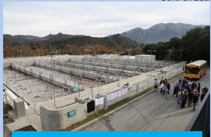
Tapia’s New Diffusers Shown Here in the Biological Nitrogen Reduction Basins
