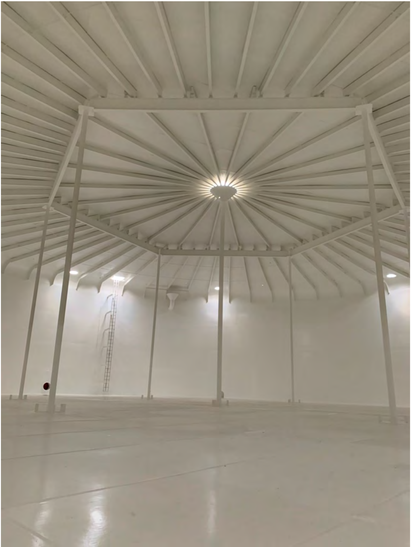
Figure 5: Cordillera Tank interior recoating complete.
