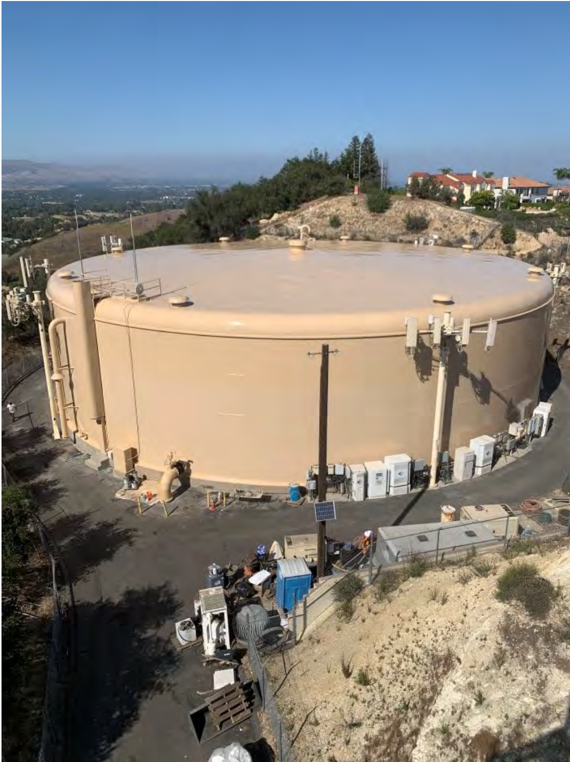
Figure 4: Cordillera Tank exterior, recoating complete
