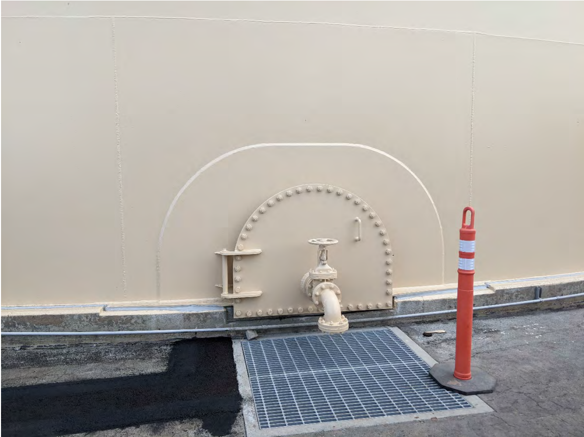
Figure 3: New clean out door installed
