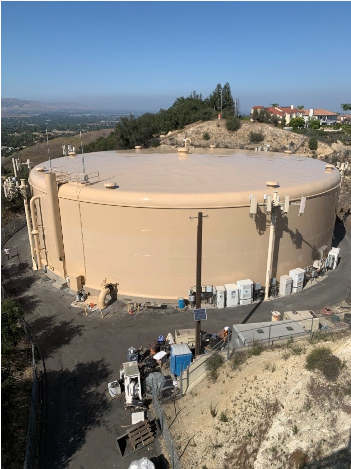
Figure 4: Cordillera Tank exterior, recoating complete
