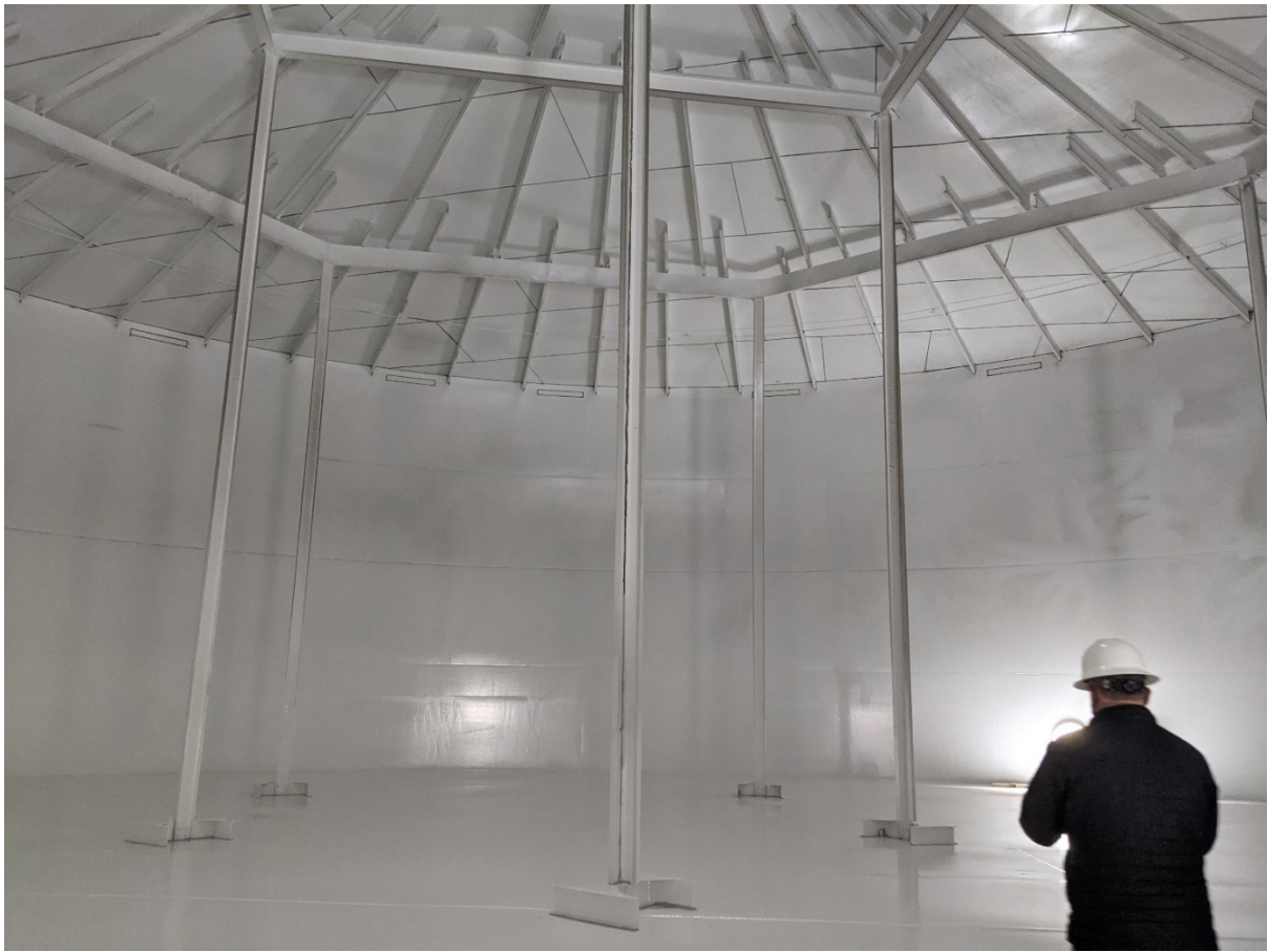
Figure 2: After picture – Saddle Peak Tank interior, recoating complete
