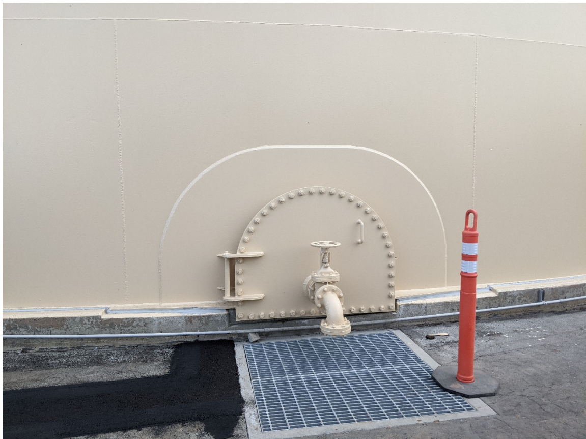
Figure 3: New clean out door installed
