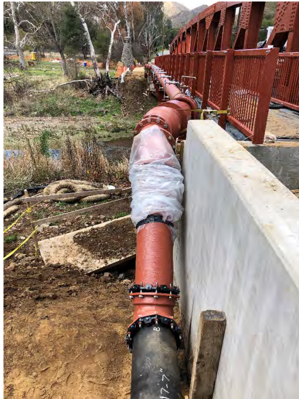
Figure 2 – Reroute of the pipe alignment around the retaining wall.
