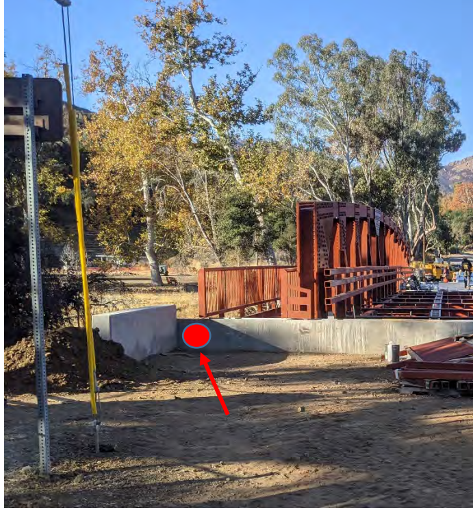
Figure 1 – Location where the pipe penetration was requested.
