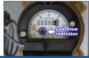
The low flow indicator will spin if any water is passing through the meter, showing when there may be a possible leak on your property.
