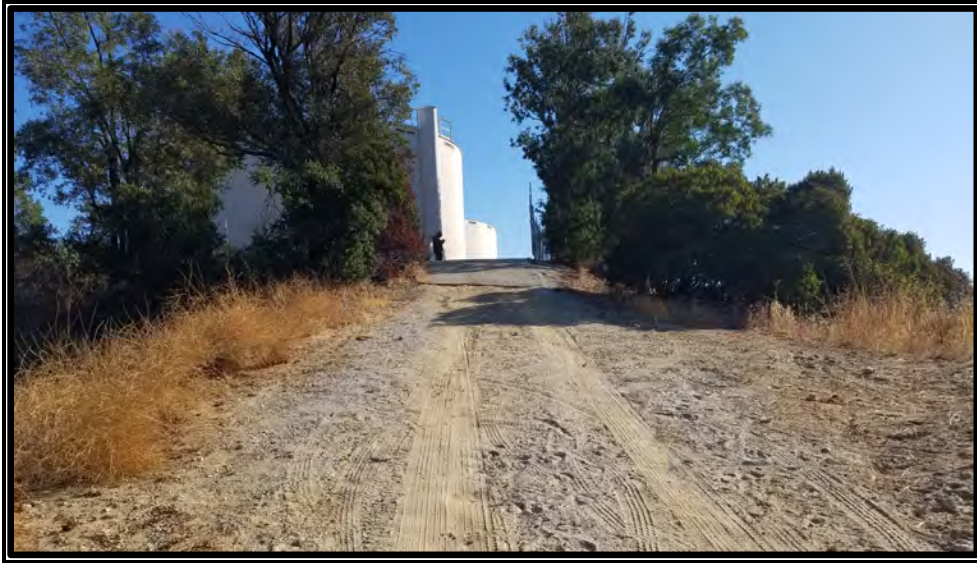
Figure 10: The Project development footprint, showing the road up to the Water Tank.
