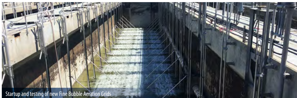
Startup and testing of new Fine Bubble Aeration Grids
