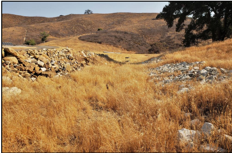
Figure 12: The modern flood control channels and basin, located at the head of the valley, which was added to control yearly flood events (originated north).
