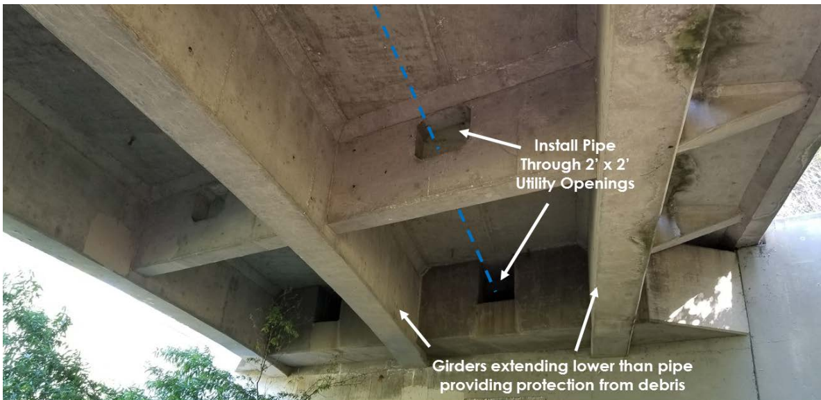
Figure 4-4 – View Under LA County Bridge: Method of Pipe Mounting
