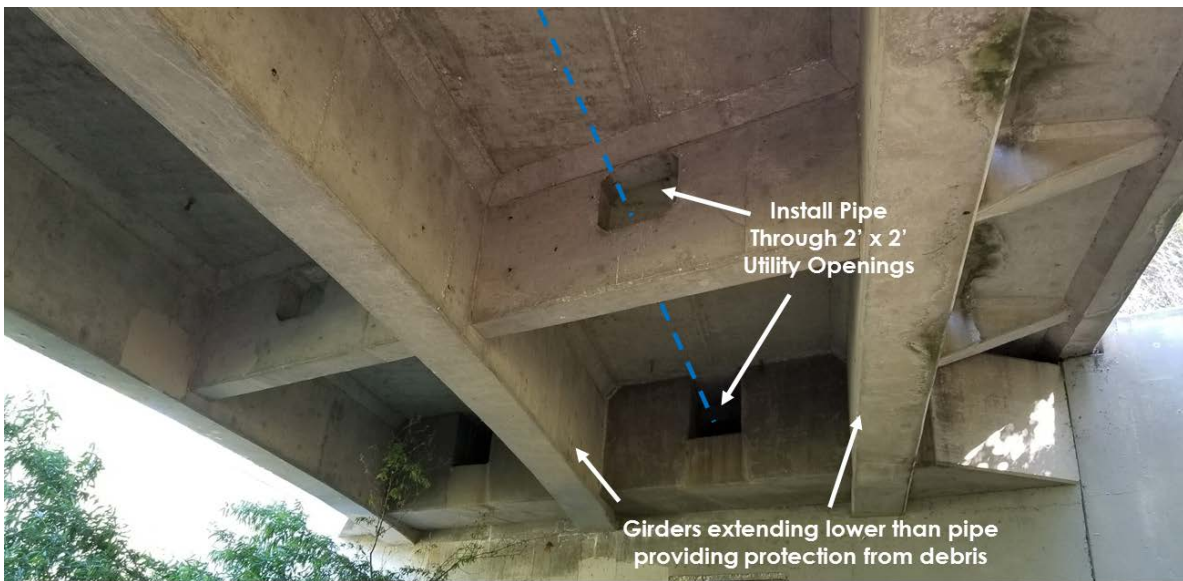
Figure 4 View Under LA County Bridge: Method of Pipe Mounting
