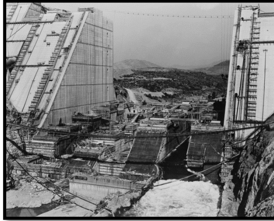
Shasta Dam under construction, 1943
